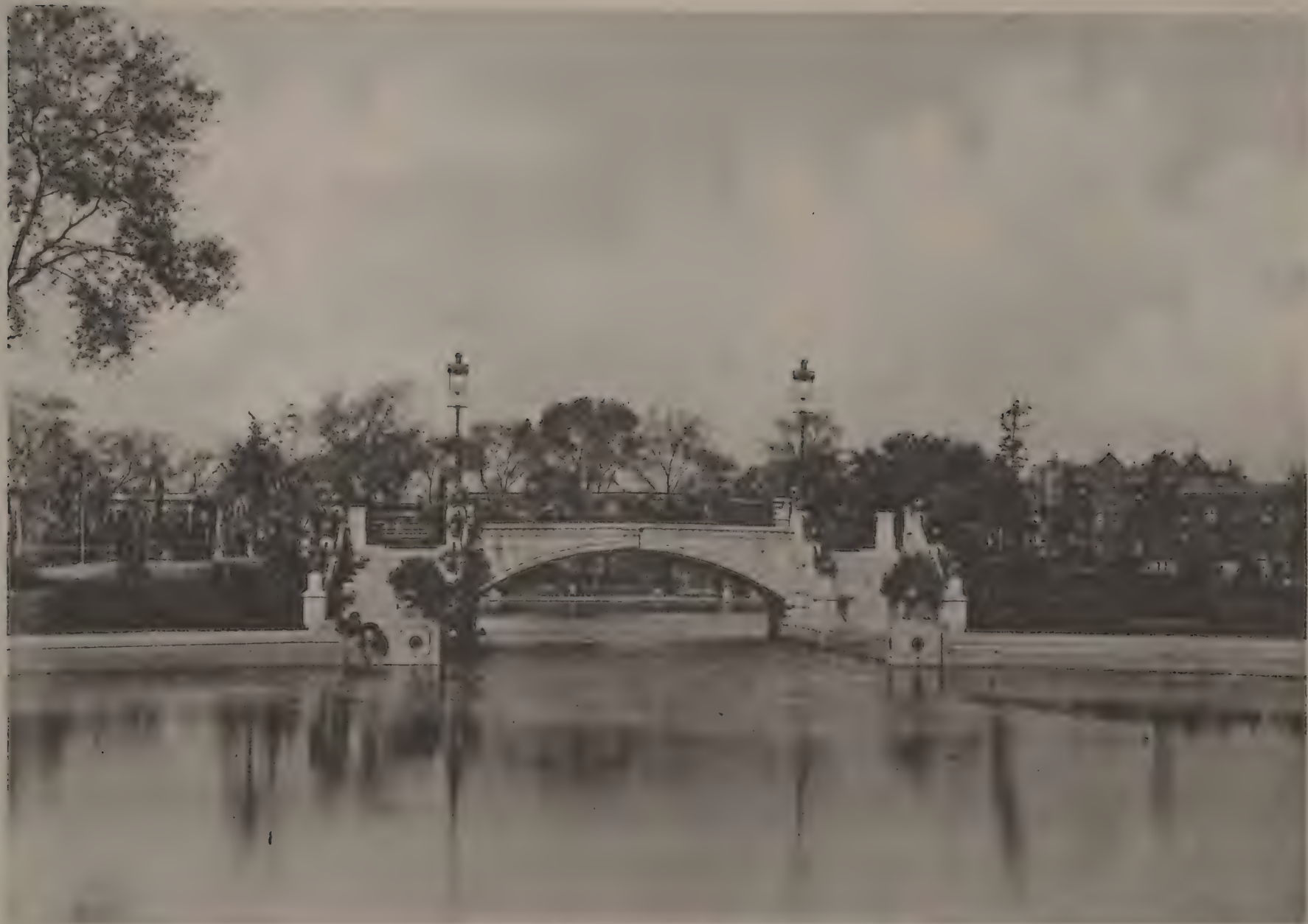
BRIDGE IN UNION PARK.
